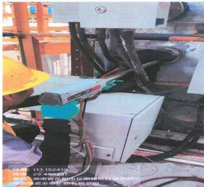
DA001 粉尘排气筒
